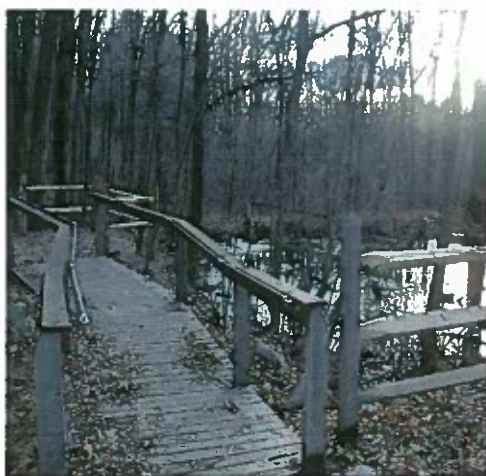
Scout James Kinicki installed new fencing surrounding the farm pond last fall.
